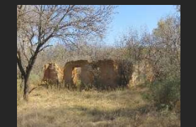
One of the buildings left over from the times when mining active – Photo by Horst Müller
